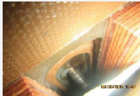
*Figure 1: Loose nut on PA core leg phase 1*
