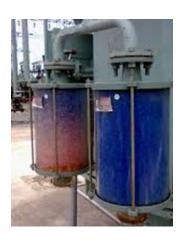
Liquid preservation systems limit the exposure of the transformer insulation structure to the atmosphere while allowing thermal expansion and contraction of the liquid due to load and ambient temperature variations. These liquid preservation systems are:
