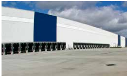
Example of Freeplan XT ® SFRC 'jointless' floor slabs
