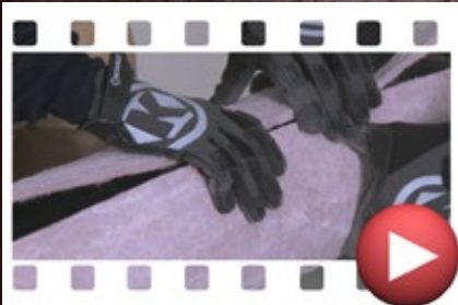
Pyrogel Insulation installation
