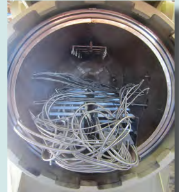
Cables in FAI LOCA Chamber
