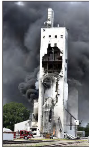
Grain Silo Explosion
