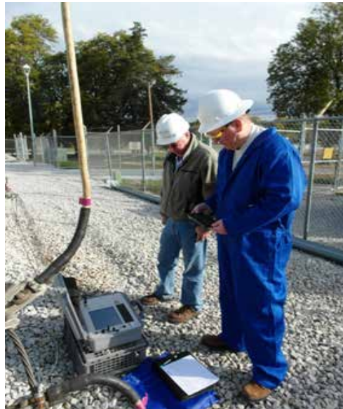
LIRA Testing of an Underground Electrical Transmission Circuit
