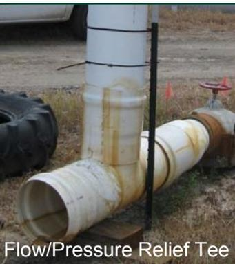
Water flow into the polytube can possibly increase during pumping. This can occur when the RPM of the power unit increases or another water outlet within the pumping system is suddenly closed.
