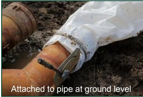
Leaking or ripping near the connection point is usually caused by the polytube flapping or fluttering.
