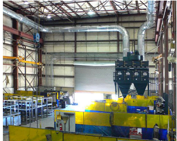
Recirculating cartridge dust collection system in Jonesboro facility.
