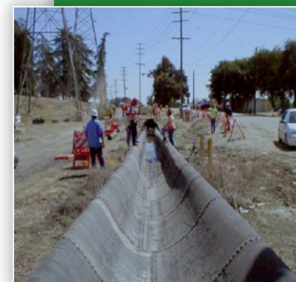
Pipeline collapse (not a canal)
