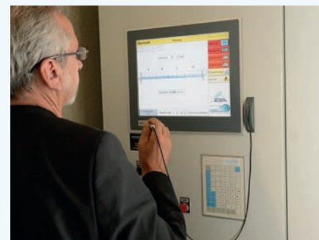
Commissioning of rubber dam
