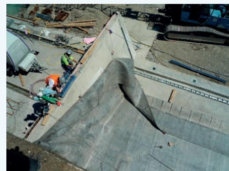
Installation of membrane
