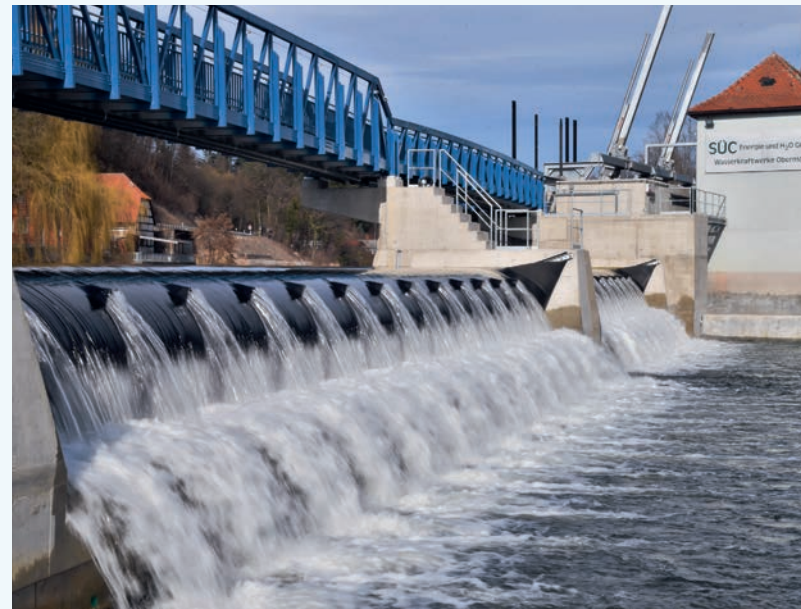
Hausen Weir / Main Germany
