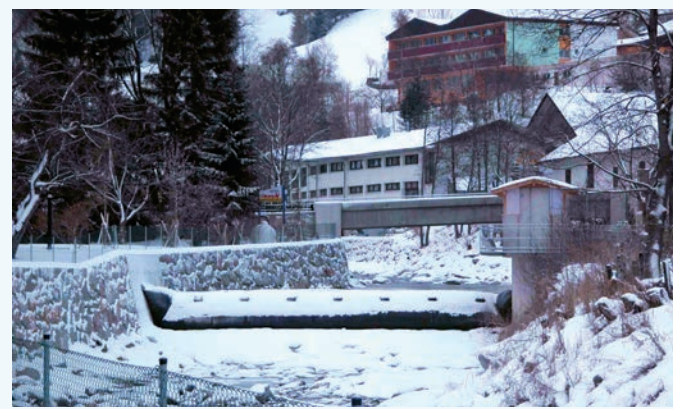
Rubber dam Steinach/Sill river Tyrol in winter time
