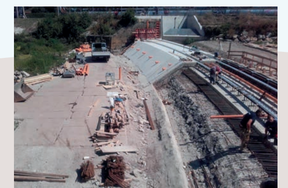
Rubber Dam Gera / Construction Phase 2016
