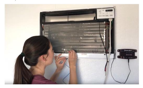
• Install one of the temperature sensors with the blue cable and black tip into the small gap by gently sliding the sensor in place ¼" only. Route the cable sensor to allow for replacement of the air conditioner front grill without pinching the cable. Plug the temperature sensor cable into the "Fins" port on the CoolBot.
