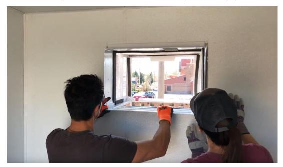
• Screw the housing to the wall with two wood screws. Make sure the cabinet tilts down at least 1/2" in the back. The weight of the air conditioner is usually sufficient to ensure 1/2" of tilt - if not shim up the front to achieve the recommended tilt.
