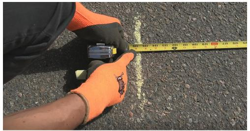
• Swing an arc 96" from the front right corner for the back right corner.
