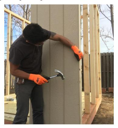
• The siding will be **flush with the second top plate (from top to bottom)** and the bottom part of the siding may hang down past the bottom plate. Leave the last TOP PLATE free to be able to nail the front and back siding after the roof is installed
