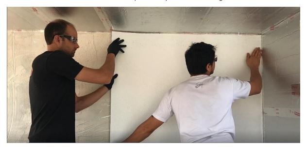
• Install FRP center and corner strips between the FRP panels.
