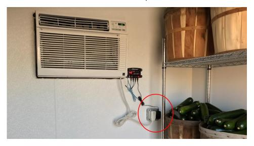
We recommend surface mounting all electrical boxes inside of the cooler to minimize compromising the insulation integrity and to reduce the chance for condensation within the electrical box.
