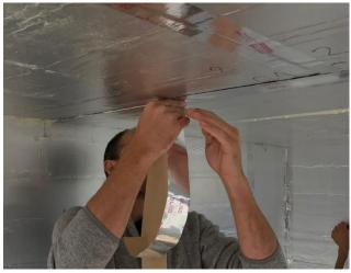
• After allowing sufficient time for the adhesive to fully cure on the first layer, cut and dry-fit a second layer of insulation to go over the first one. NOTE: DO NOT match the seams of your first layer. Install your second layer staggering the seams when compared to the first layer.
