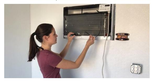
Install the Heater Cable by laying the red tip and air conditioner temperature sensor alongside
