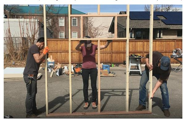
• Note that the top double plates on the back and front wall overlap the top plates on the left and right walls.
