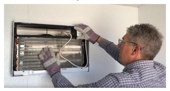
• Replace the screws that hold the housing and the air conditioner together.
