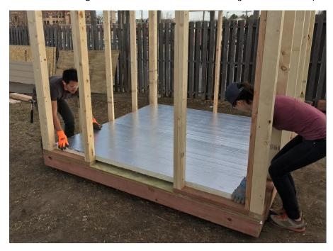
Once your insulation is in place, cut and fit ¾" treated plywood panels to close your floor.
