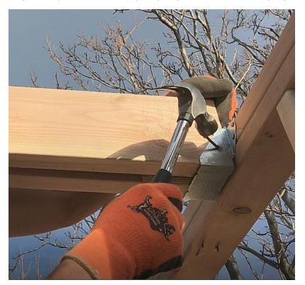
• In order to support the ceiling light, we will install a 2 by 4 support. Measure the distance between the double joists and cut a 2 by 4 to this length. Nail the 2 by 4 between the double joists centered from front to back of the cooler.
