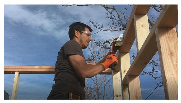
• Place the double joists into the double joist hangers.
