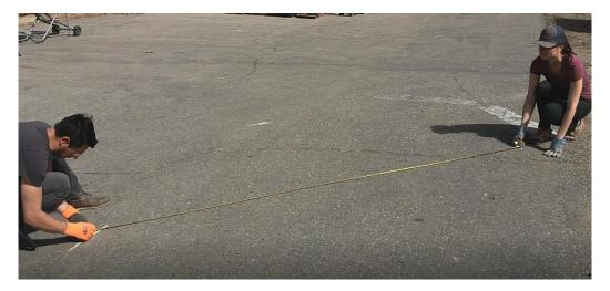
• Snap chalk lines from the arc intersections to mark the perimeter walls of your cooler.
