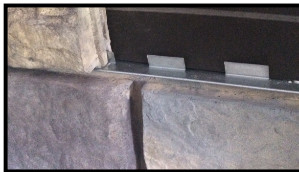
Clearances Gap 3/8”-1/2” at all openings. Do not install tight against other materials
