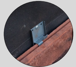
Standard Galv. Clip Minimum 2 clips per square foot
