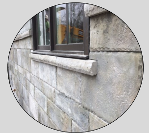
Clearances Gap 3/8”-1/2” at all openings. Do not install tight against other materials
