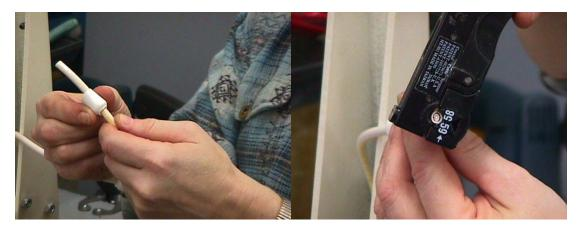
• Install connectors then use the crimpier to secure the connectors
