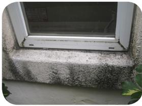
**Caulking around openings:** Caulking around exterior doors and windows can become mildewed or cracked from summer rains and the hot Florida sun. This often leads to claims from water intrusion, not just in a hurricane, but any large rain event. The lack of a watertight seal
