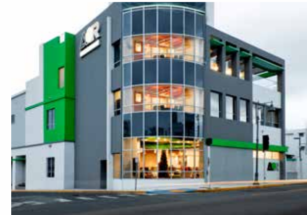
AOR Building Supplies
