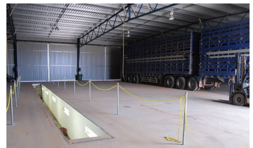
Floor Service Pit
