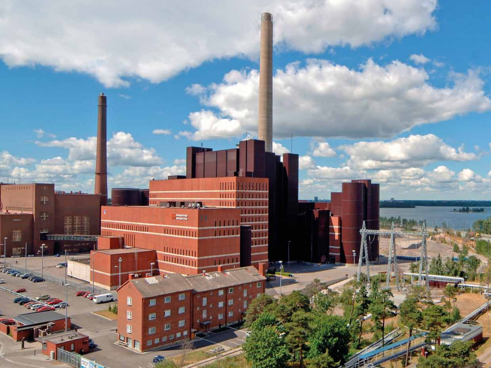
FIGURE 2. The on-line monitoring system is in use at the Helsingin Energia's Salmisaari Power Plant.
