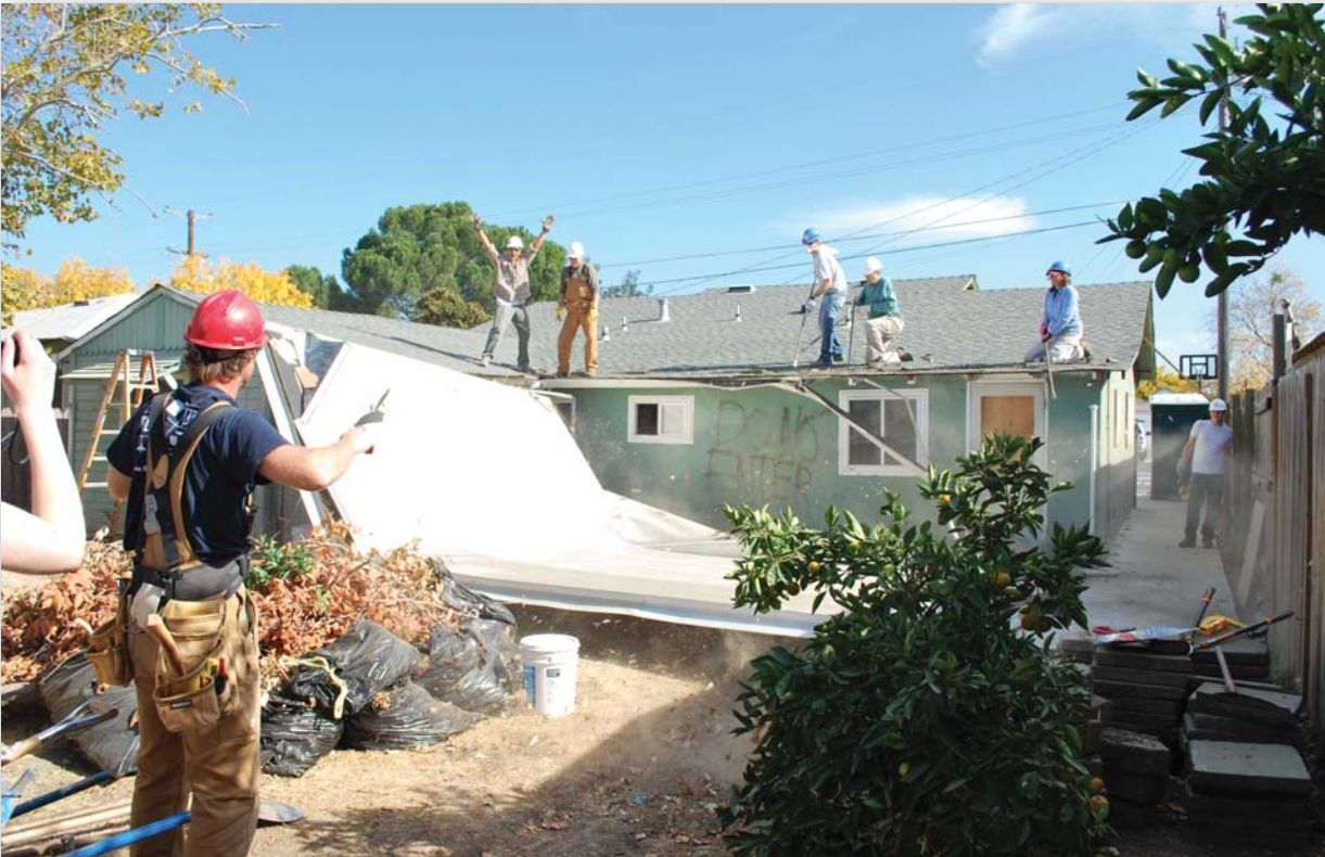
THE OUTDOOR CREW CHEERS after safely collapsing the outdoor patio roof. The actual collapse took just a few minutes, preceded by hours of prep work to unmoor the roof and ensure that it fell straight down.
