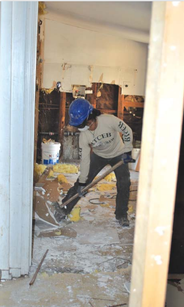
THE INSIDE CREW had the messy task of removing all of the interior wall board, doors, fixtures, insulation, and trim. "Everyone seemed ready to get their hands dirty while still maintaining a safe work environment," comments Tina Chou, shown here attacking some dry wall.
