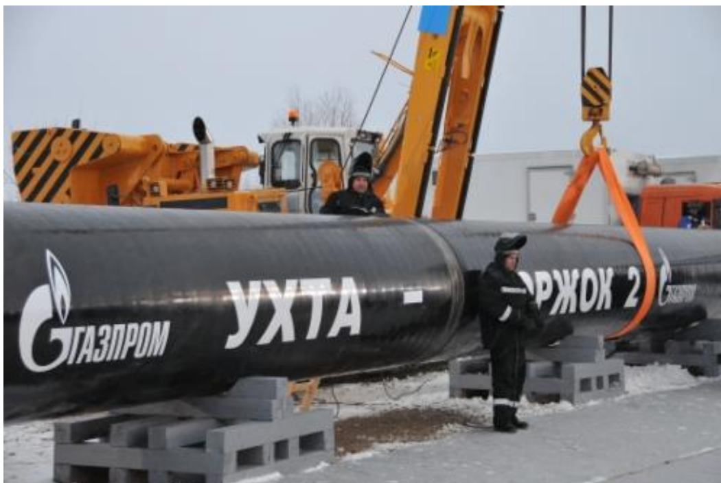
Figure 4-7: Construction of a onshore pipeline (Gazprom, 2016)
