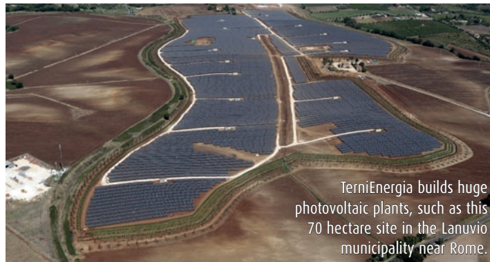
TerniEnergia builds huge photovoltaic plants, such as this 70 hectare site in the Lanuvio municipality near Rome. ranging from 195 to 240 hectares, and are being constructed for an unnamed major Italian utility firm.
