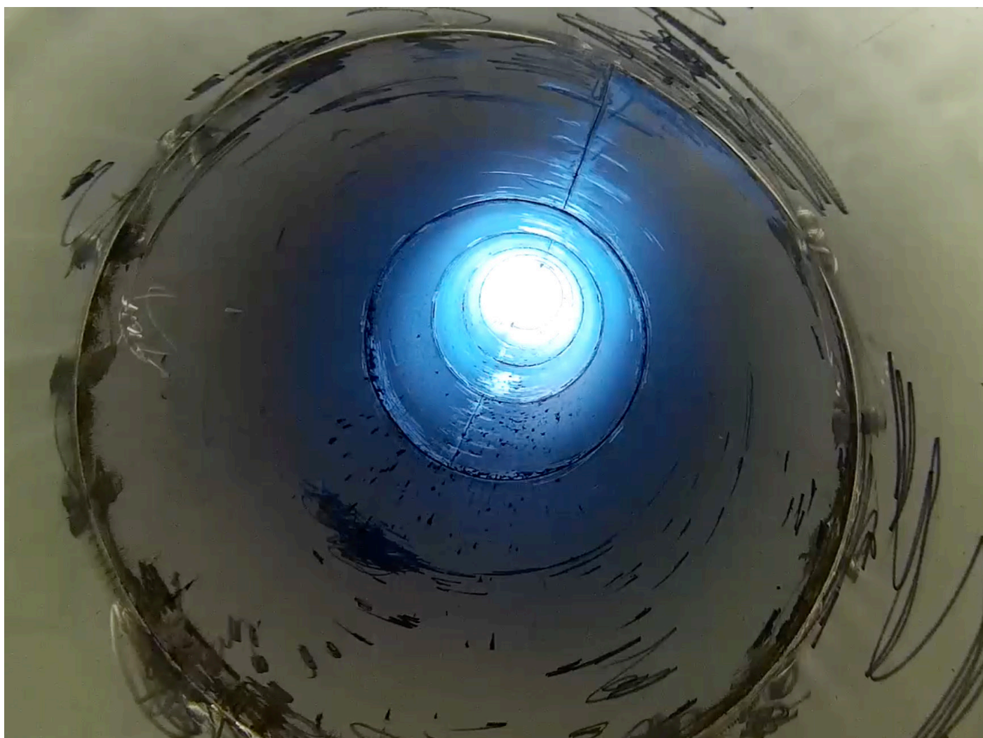
Picture from an Elios 2 Inspection of a Stack
