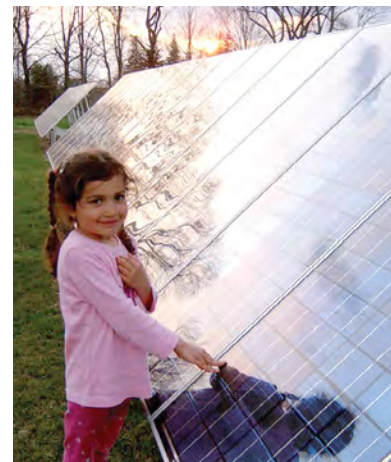
Backyard solar array in Andover, Mass.
