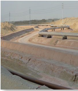
Pre-insulated Pipe Facilitated Construction
