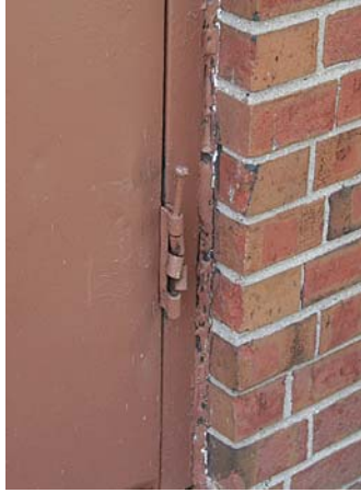
Damaged hardware on exterior door
