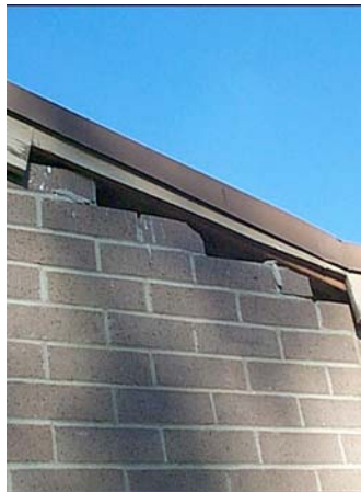
Damage creates potential for water penetration
