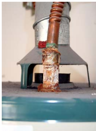
Significant corrosion and rust damage
