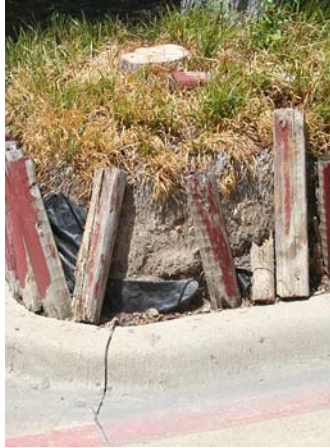
Retaining wall is leaning and falling
