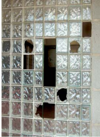
Holes in wall penetrate completely
