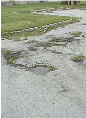
Potholes and loose material
