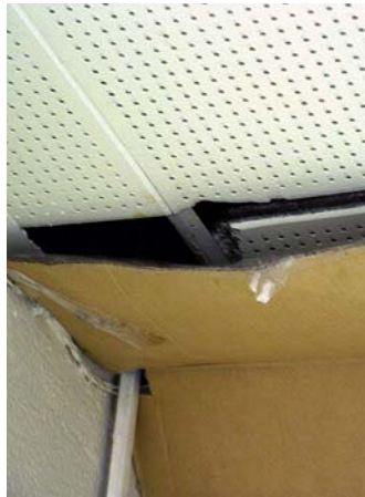
Significant buckling of ceiling
