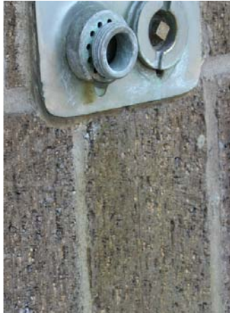
Water leaking from central water supply
