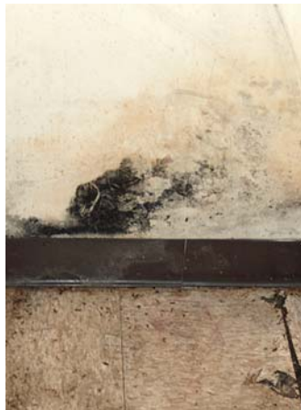
Surface substantially damaged by mold
