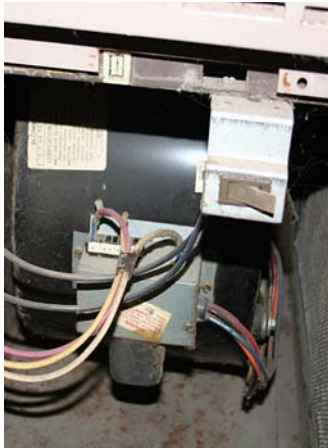
Broken motor on HVAC system – non-operational
