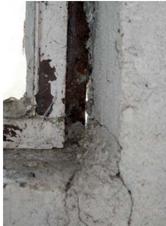
Significant damage to seals results in window leaks
