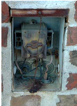
Exposed electrical connections
