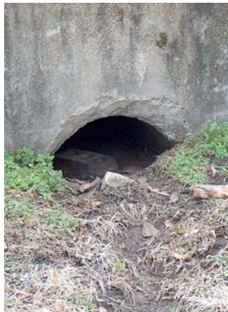
Obstructed storm drain
