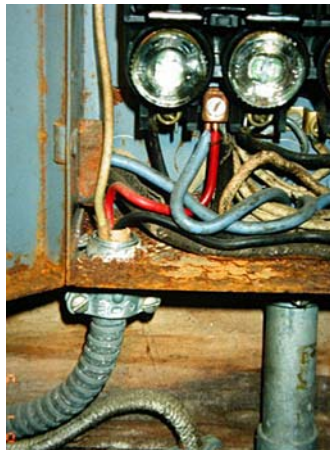
Corrosion on electrical enclosure
