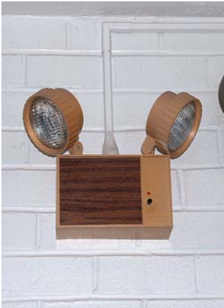
Auxiliary lighting is non-functional
