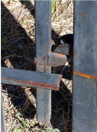
Exterior fence hinge is broken
