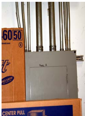
Electrical panel is inaccessible
