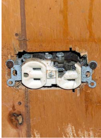
Outlet missing coverplate
