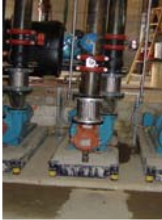
Boiler pump leaking
