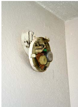
Smoke detector is non-functional
