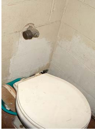
Toilet cannot be flushed due to missing tank
