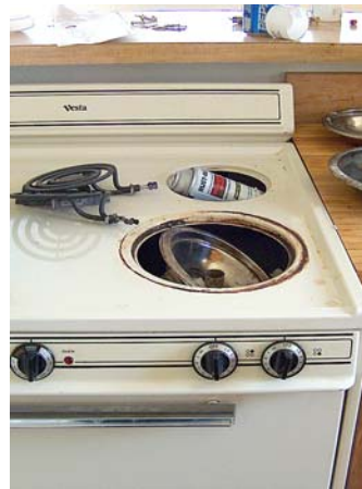
Two burners on stove top are non-functional
