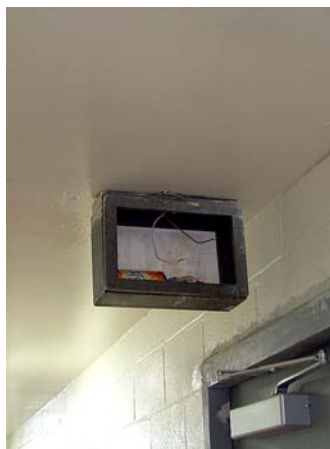
Exit sign missing, cannot be illuminated
