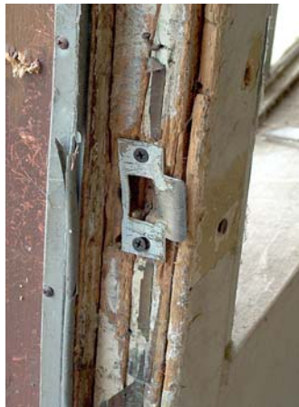
Damage to frame prevents door from functioning normally
