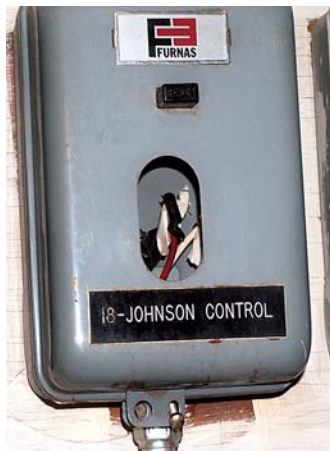
Exposed electrical connections
