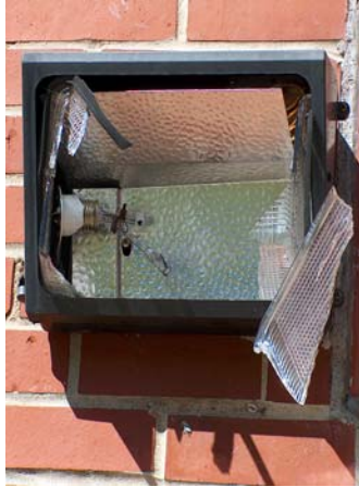
Broken exterior light
