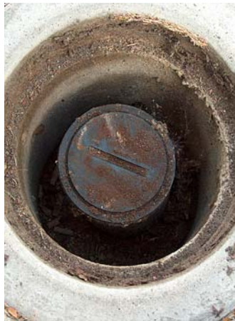
Missing manhole cover
