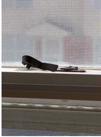
Window lock is non-operational, window cannot be secured
