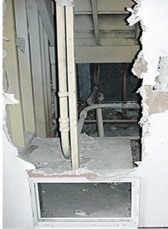
Hole penetrates to adjoining room
