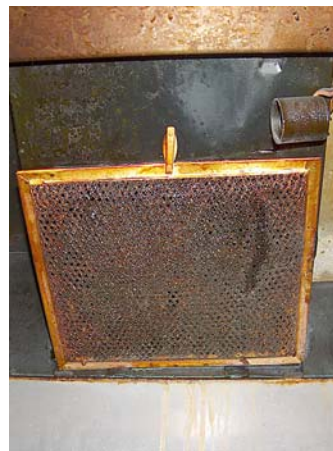
Accumulation of dirt renders exhaust fan non-functional
