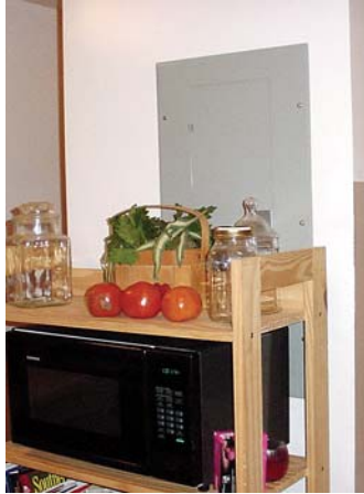
Electrical panel inaccessible in emergency
