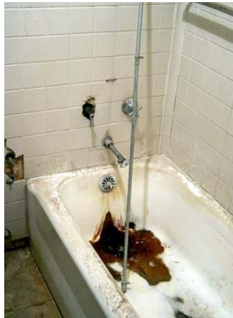
Extensive damage has rendered tub unusable
