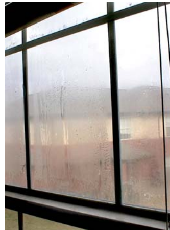
Failed Thermopane
