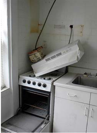
Range exhaust fan is inoperable
