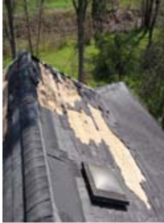
Shingles missing more than 2 squares
