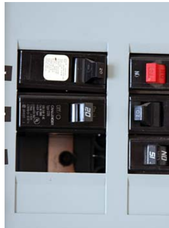
Open breaker ports
