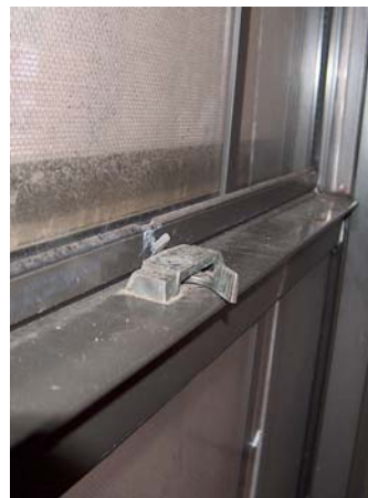
Lock not functioning, window cannot be secured
