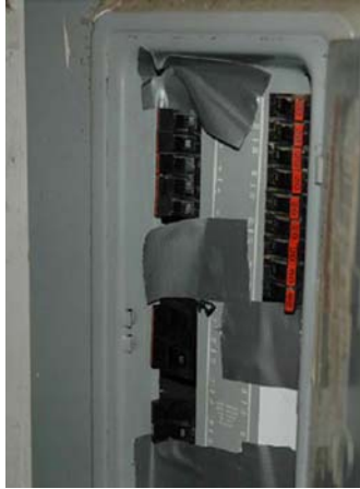
Missing breakers not appropriately blanked-off
