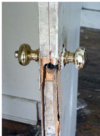
Damaged hardware renders door unlockable
