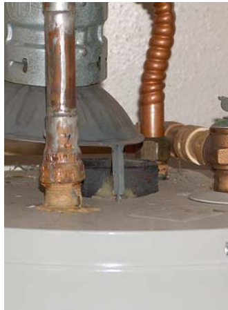
Misaligned chimney on hot water heater
