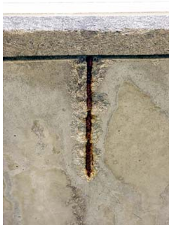
Foundation spalling exposed rebar
