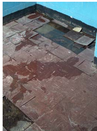
Substantial water damage to floor
