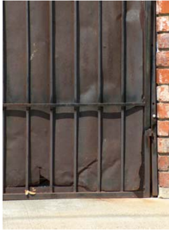
Security door is nonfunctional
