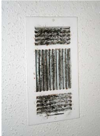
Mold apparent around air vent
