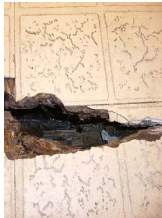
Deteriorated Subfloor
