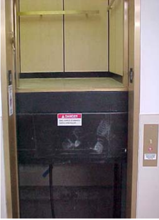
Doors open when car is not in proper position
