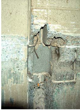
Exposure of reinforcing material
