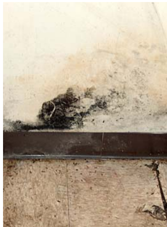
Wall substantially damaged by mold
