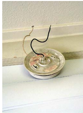
Smoke detector non-functional
