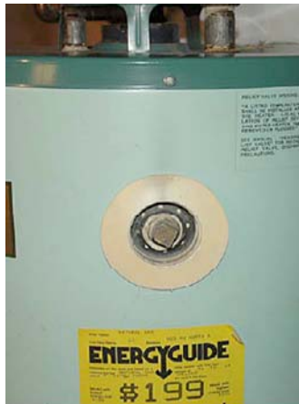
Missing pressure relief valve
