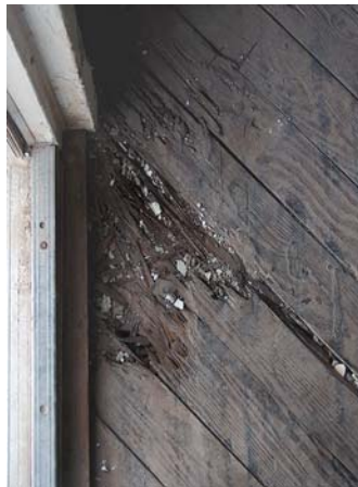
Large area of subfloor damage
