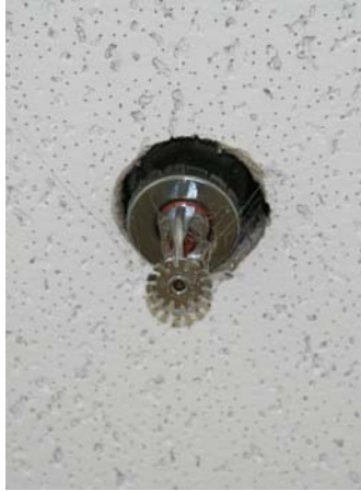
Missing sprinkler head or its components
