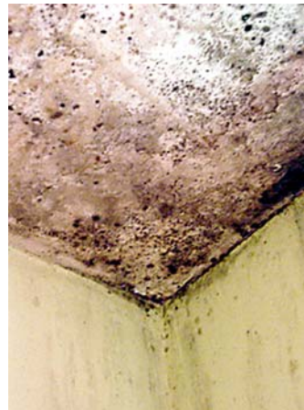
More than 50% ceiling area affected by mold
