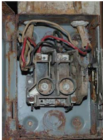
Evidence of leaks and corrosion
