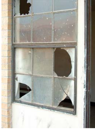
Multiple broken glass panes
