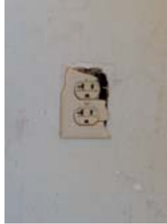
Broken outlet coverplate
