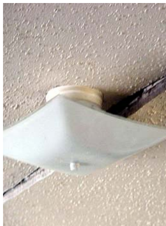
Ceiling damage – Sagging
