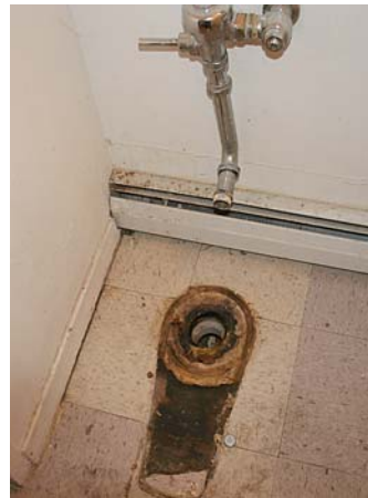
Toilet has been removed from bathroom
