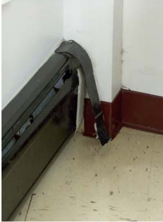
Cover compromised on radiant heat system
