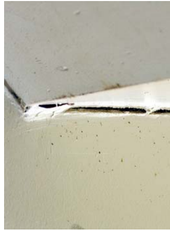
Crack greater than 1/8 inch wide and 11 inches long
