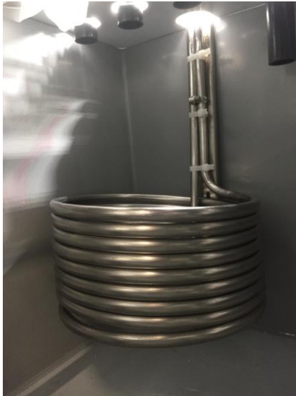
Stainless Steel Cooling Coil installed in reservoir
