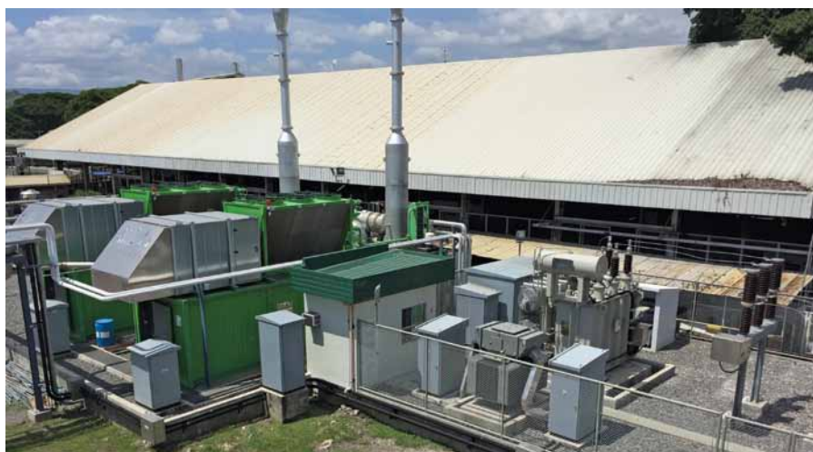
The generator sets for the waste-to-energy facility
