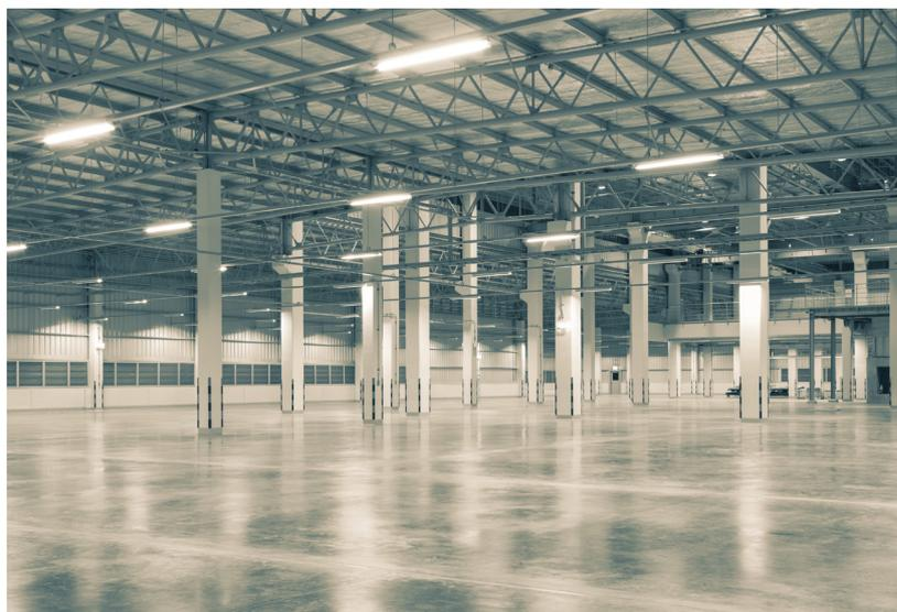
The reinforced concrete slab must be made with expansion joints, in order to prevent cracking and should be covered with a cement cap a few centimetres thick, which is rendered smooth and hardened (to prevent powdering).
