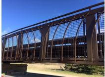
derived from the shape of the nearby Conservatory. The single span was delivered to the site and lifted into place via crane, and the bridge opened to the public just one week later.
