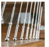
Bevelled washers are used on stair sections where a tensioner and rod terminal are used
