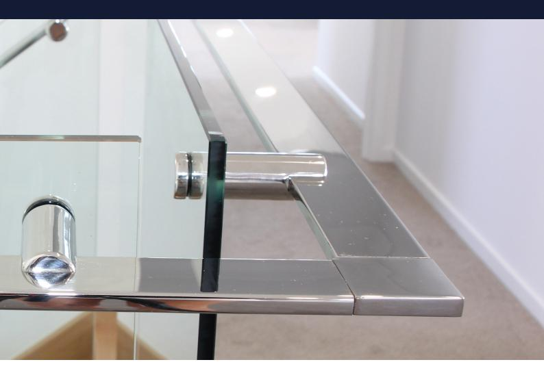
Handrail Brackets for mounting to the side of a wall are available in a range of sizes and designs suitable for supporting timber and stainless steel handrails. Some brackets can be fitted to wall or glass panels. All brackets are available in mirror polish or satin finish.
