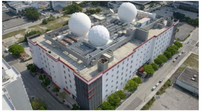
2001: The Network Access Point (NAP) of the Americas in Miami, built, owned and operated by Terremark, eventually sold to Verizon in 2011 for $2 Billion.
