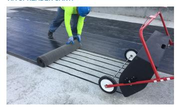
When using the spreader cart to apply COLPLY EF in ribbons, 3/4" to 7/8" inch holes should be predrilled for the required spacing (12" o.c., 6" o.c., etc.). With the cart laying down, up to four pails of COLPLY EF can be loaded into the tank at one time (20 gals). With an application rate of 1 gallon per square, 1 full tank will cover between 15 and 20 squares.
