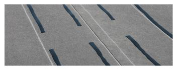
Once the adhesive is applied in ribbons, the membrane must be immediately applied. After rolling out the membrane into the adhesive, a weighted roller should be used over the entire surface of the membrane. The weighted roller is critical to ensuring proper bead width of  $2\,\%$ " to 3" beneath the membrane.
