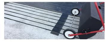
After 30 to 45 minutes of application (may be less based on heat and humidity), any adhesive left in the tank will begin to skin over. Once this happens, this tank cannot be refilled and must be swapped out for a new tank. Multiple tanks should be kept on site at all times.
