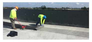
To apply, simply turn the cart over and begin walking in the direction the membrane will roll out. Be sure to maintain the proper bead size of  $\frac{1}{2}$ " to  $\frac{3}{4}$ " while applying. Every 33 to 45 feet, a six inch horizontal break must be provided to allow for cross venting between channels.
