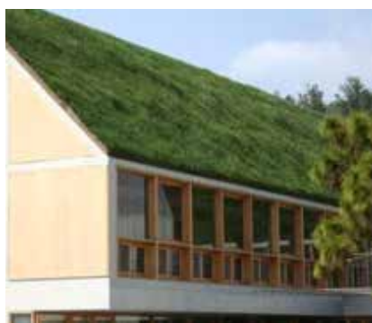
Green roof insulates and controls stormwater runoff
