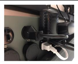
1. Unplug front or rear control box power cable from the Power Bar mounted underneath the rear table or on the side of the CPU cabinet. Need to wait a full 30 seconds for all power to drain from control box.
