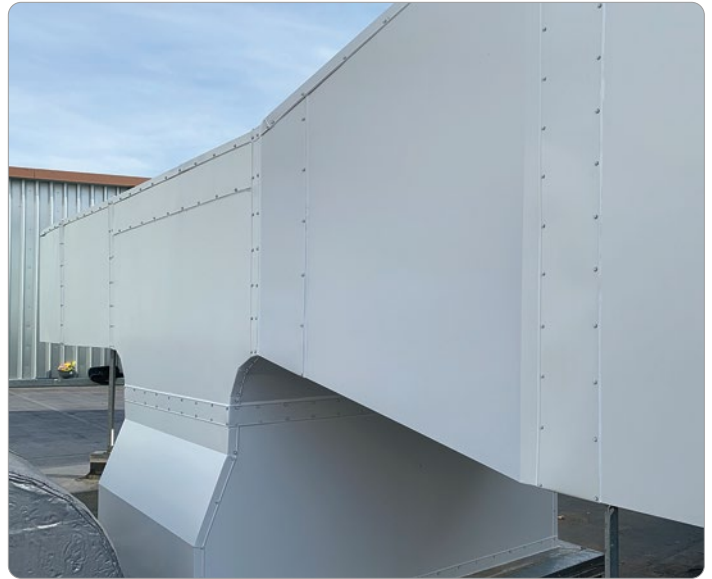
Techna-Duc® is used to insulate exterior HVAC ducts. Insulation panels are custom fit and prefabricated to enclose ductwork with a weathertight seal.
