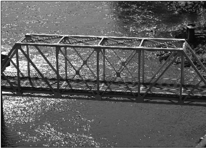
A steel truss bridge. Photo courtesy of MorgueFile.com.
