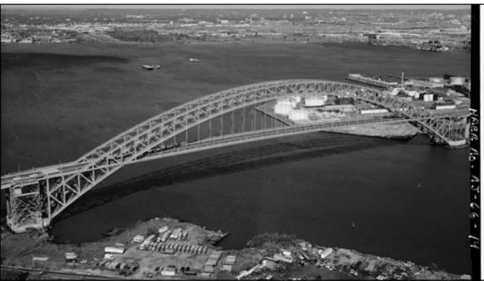
The Bayonne Bridge in New Jersey is a steel arch bridge, though it also incorporates elements of truss and suspension bridges. Photo courtesy of The Library of Congress.
