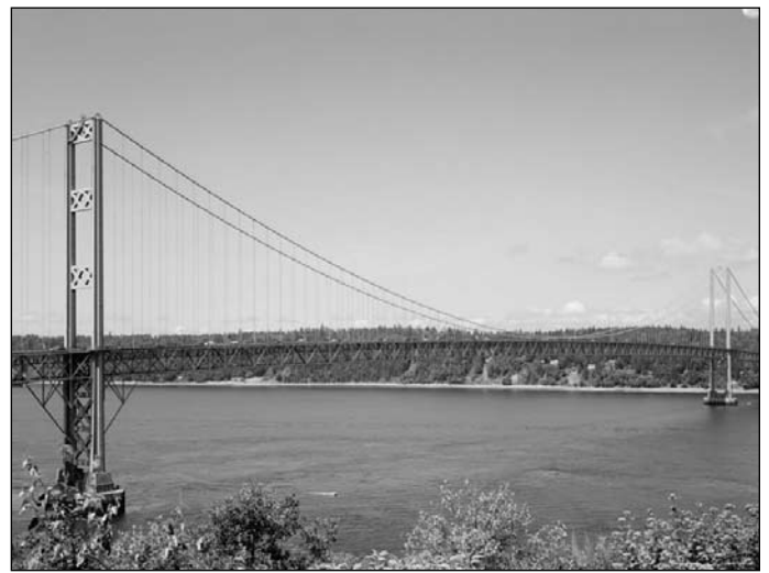
Bridges must be built to withstand the environment as well as traffic. This bridge over Tacoma Bay in Washington State (shown completed above) was destroyed by a 42 mph wind (below). Examples like this illustrate the importance of good engineering. Photos courtesy of The Library of Congress.
