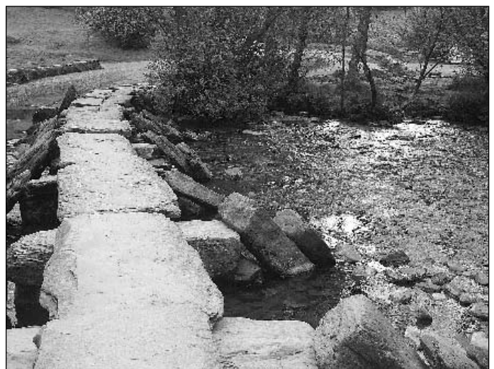
Tarr Steps, the clapper bridge over the River Barle, is said to be the oldest bridge in Europe. Photo courtesy of MorgueFile.com.
