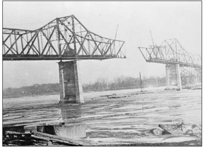
This photo of the MacArthur Bridge, built over the Mississippi River between Iowa and Illinois, demonstrates how the ends of a cantilever bridge are built first. Then, the middle is placed between. Photo courtesy of the Library of Congress.
