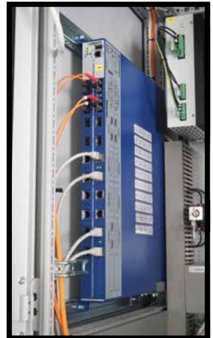
The substation used a MACH1000 Industrial Ethernet Switch in a vertical installation in the control cabinet.
