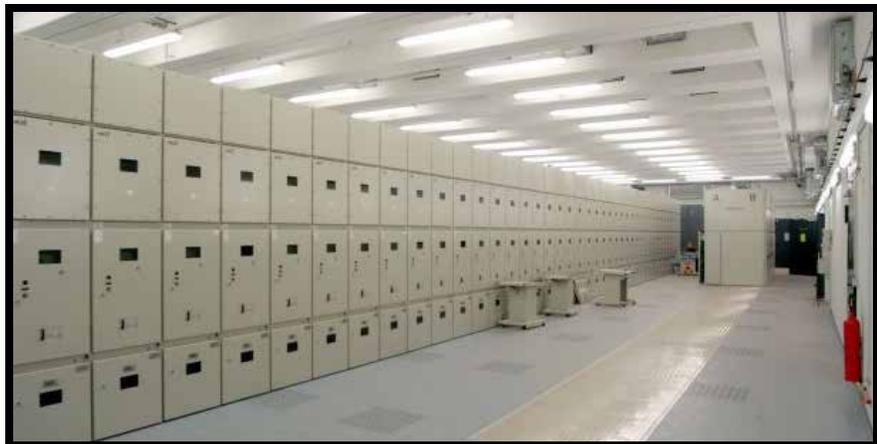
View into the depths: The 10 kV control cabinet room of the new substation is located approximately 17 meters below the surface.
