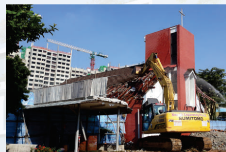
Demolition works started in December 2018
