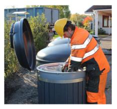
Picture 3.8 Open and straighten the lifting bag before placing it in the container.
