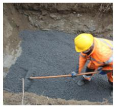
Image 3.1. 50 mm of 0-16 mm crushed gravel can be used for levelling.
