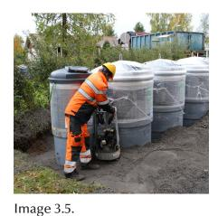
Ballast material is then placed on top of the crushed stone (anchoring). Use a spirit level to ensure the container is straight and level.
