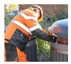
Picture 3.7 Remove the lifting loops.
