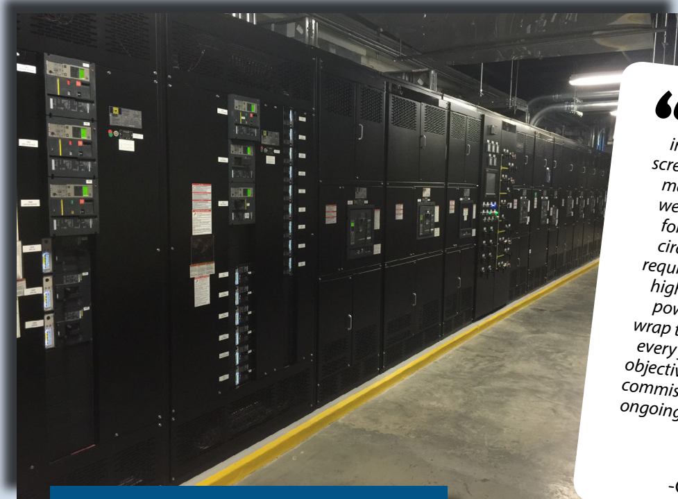
Typical DVL intelligent switchgear installation
