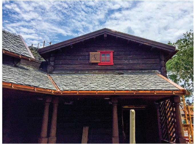
The modified roof consisted of a SOPREMA Sopralene Flam 180 three ply system.
