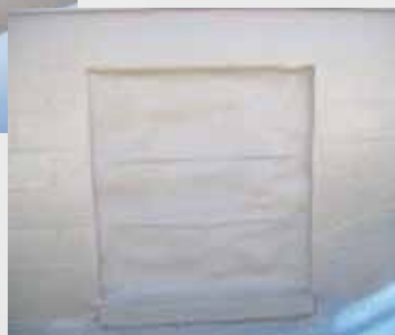
Window after spray-foam and silicone coating
