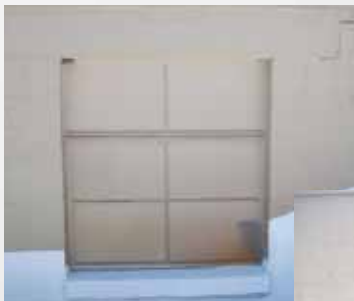
Unused window before spray-foam application
