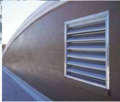
Silicone Top Coat and Restoration
