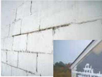
Cracks and Discoloration
