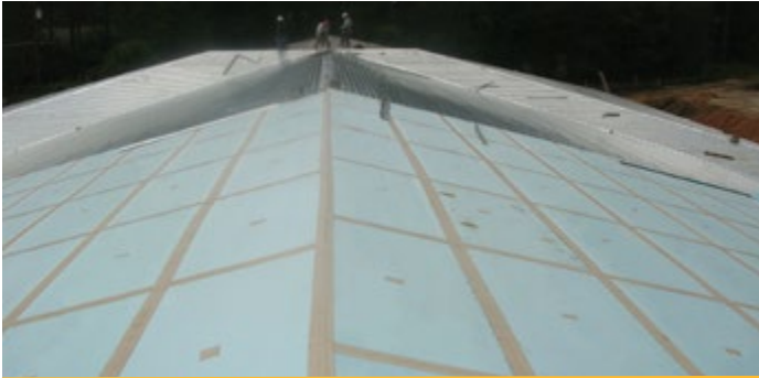
Install insulation in single or multiple layers, sealing the joints in the top layer with tape (see list of suggested tapes on page 3). If multiple layers of insulation are installed, offset (stagger) board joints between layers a minimum of 6 inches. Ask your Dow representative for additional details, or call 1-866-583-BLUE (2583).
