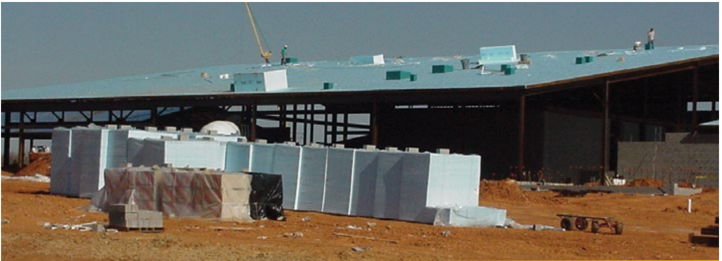
STYROFOAM™ Brand DECKMATE™ Plus Insulation can be applied directly on metal decks.
