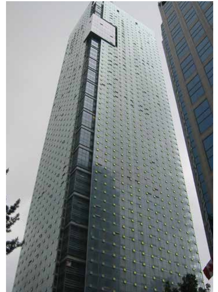
Designed by James K. M. Cheng Architects Inc., the visually stunning Living Shangri-La hotel, located on the Vancouver waterfront, was built using CURTAINROCK® and ROXUL SAFE™ products as its specified insulation.
