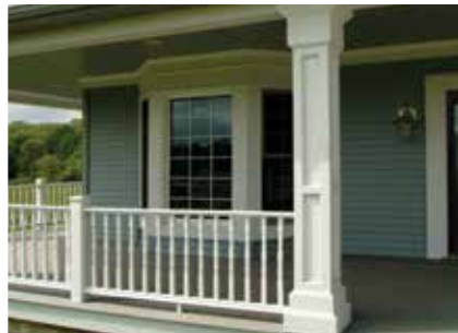
PORCH POSTS AND TRIM
