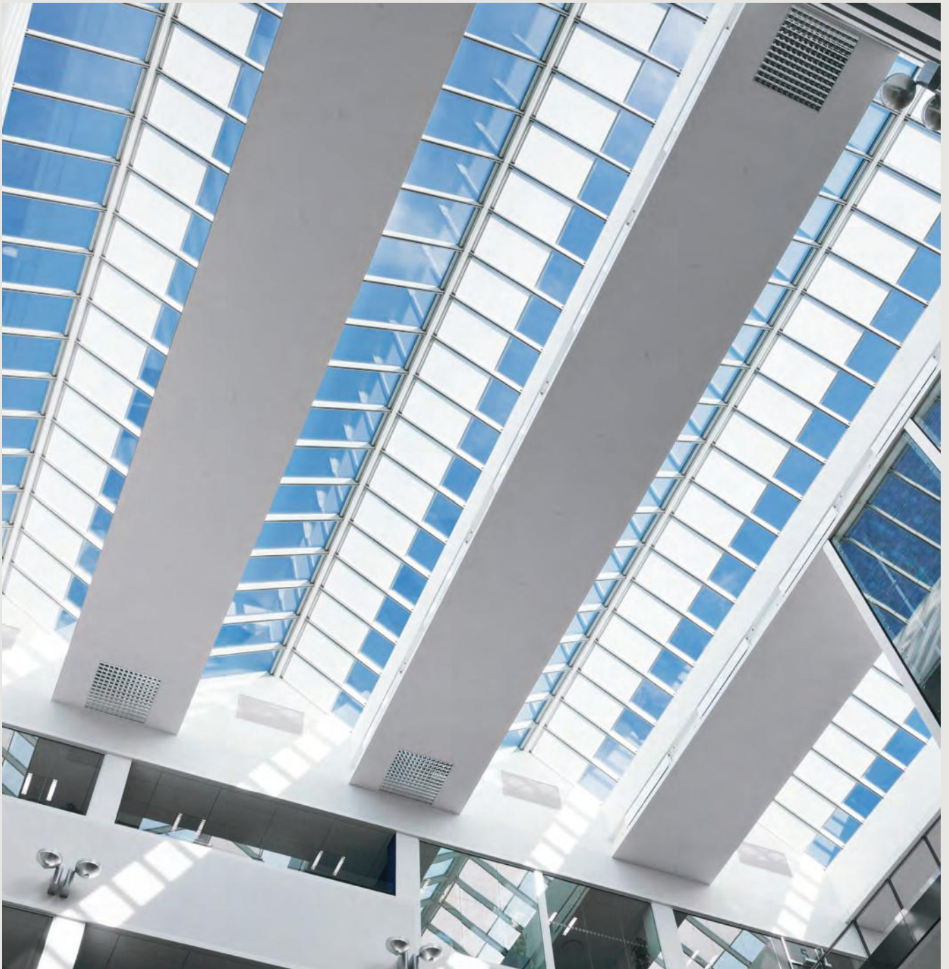
Roller shades on south facing modules in Siemens Head Office, Ballerup, Denmark
