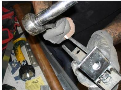
**Why the incident occurred:** The socket slipped when he was tightening the bolt causing his right finger to hit the Unistrut. The piece of Unistrut was not deburred after being cut. **The result:** Three hours in the clinic and eight stitches.
