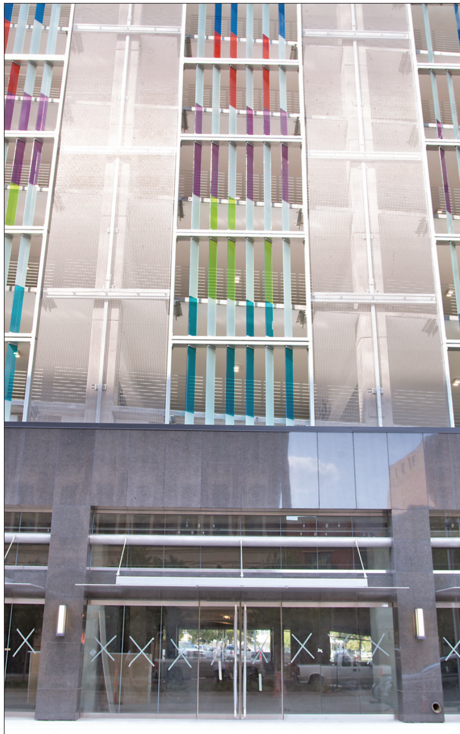
The new Arts District parking garage in downtown Oklahoma City. PHOTO BY BRENT FUCHS
