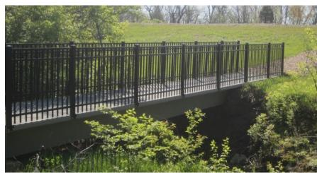
Our zero maintenance Fiberglass Reinforced Polymer (FRP) trail bridges eliminate the financial strain conventional bridge products can place on park operations budgets. Bridges need to blend with natural surroundings so our high performance products combine aesthetics with function. FRP materials provide superior strength and resist corrosion from water, salt and chemicals. Our pre-fabricated, light-weight bridges are easy to install.
