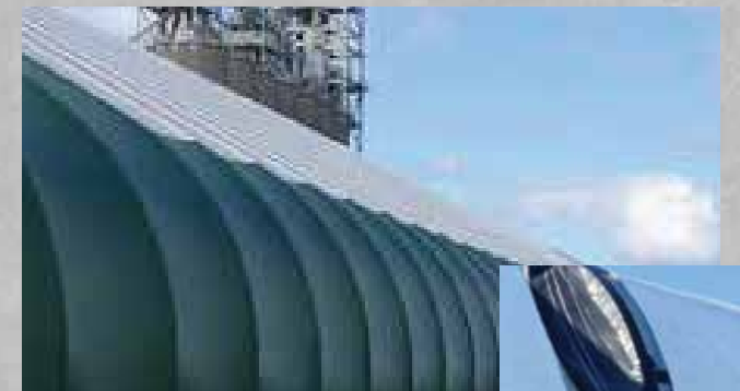
Round tube allows for proper tensioning without cover failure.
